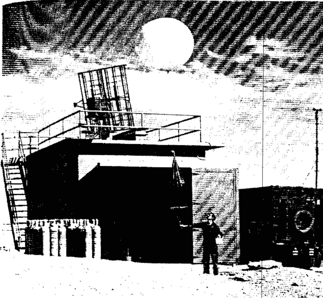
The United States Air Force weather station shown above is located near the Control Point at the Nevada Proving Ground. During continental tests, weather personnel send many helium-filled Raob (radar-observer) balloons to the upper atmosphere to check on temperatures, dew points, humidity and wind velocities. The radar tracking instrument, located on top of the test weather station, charts wind velocities and directions to determine cloud paths after detonations.
