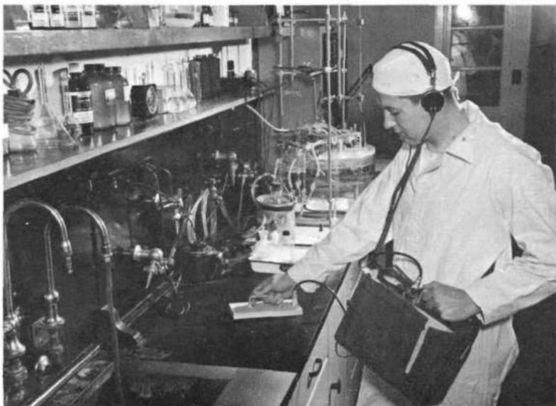
*A health monitor using a "PeeWee" (proportional alpha counter) to search for plutonium contamination during a routine survey of laboratory facilities. As little as a billionth of a gram of plutonium can be detected with this meter.*
